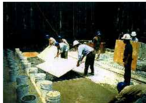
Place plywood over floor sheet
