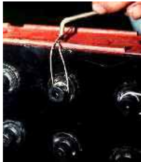
Attach tie wire to top of form
