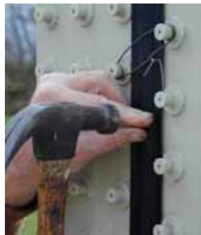
Pre-drill through center of H-Zip Strip and install finish nail
