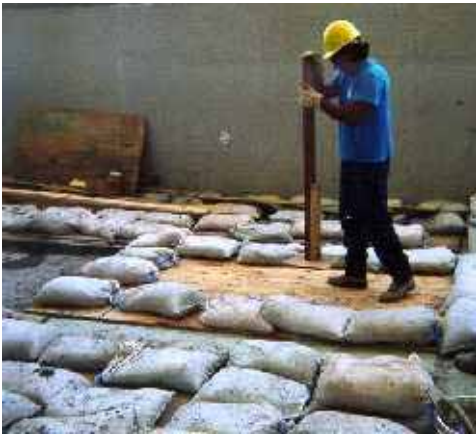
Tamp to seat anchors, do not over tamp
