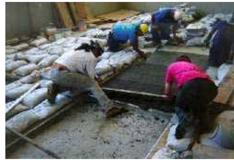
Screed sand cement setting bed
