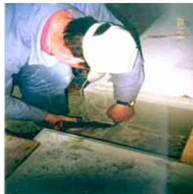
All seams thermal welded
