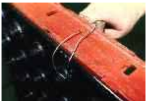
Wrap tie wire around anchor
