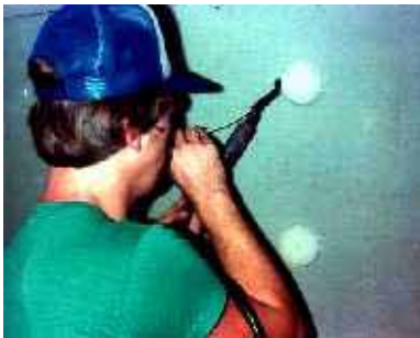
Welding of disc seal over form tie hole
