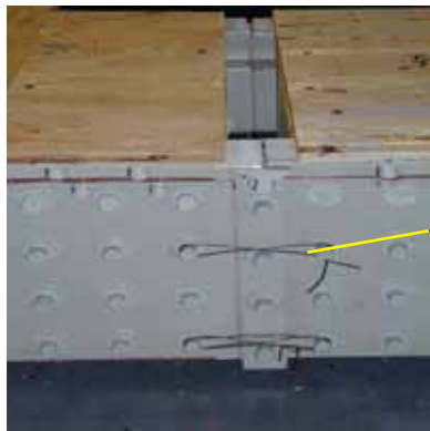
Join sections with tie wire
