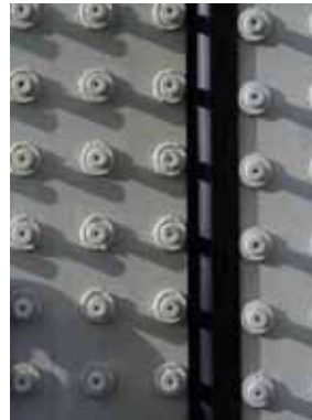
H-Zip strip joining two sheets
