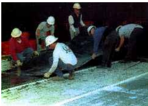
Place floor sheet over setting bed
