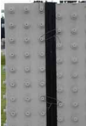
Wrap and draw tie wire across diagonal anchors
