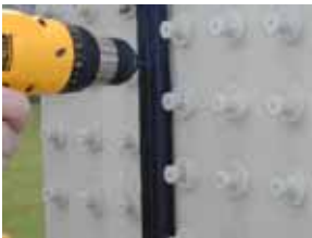
Pre-drill through center of H-Zip Strip and install finish nail
