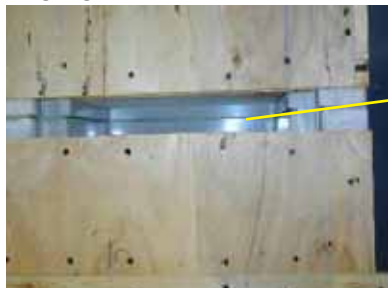
Align gap, sides and bottom
