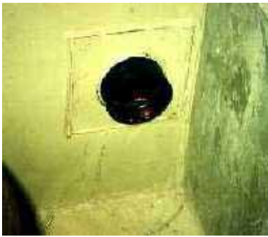
Collar over pipe welded to sheet
