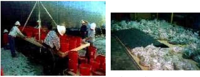
Place ballast on plywood
