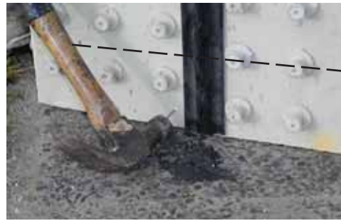
Install finish nail below Anchor-Lok floor elevation
