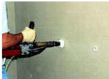
Extrusion welding of form tie hole
