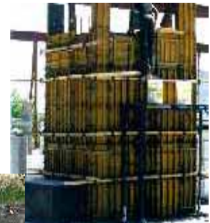
Plywood face and metal frames
