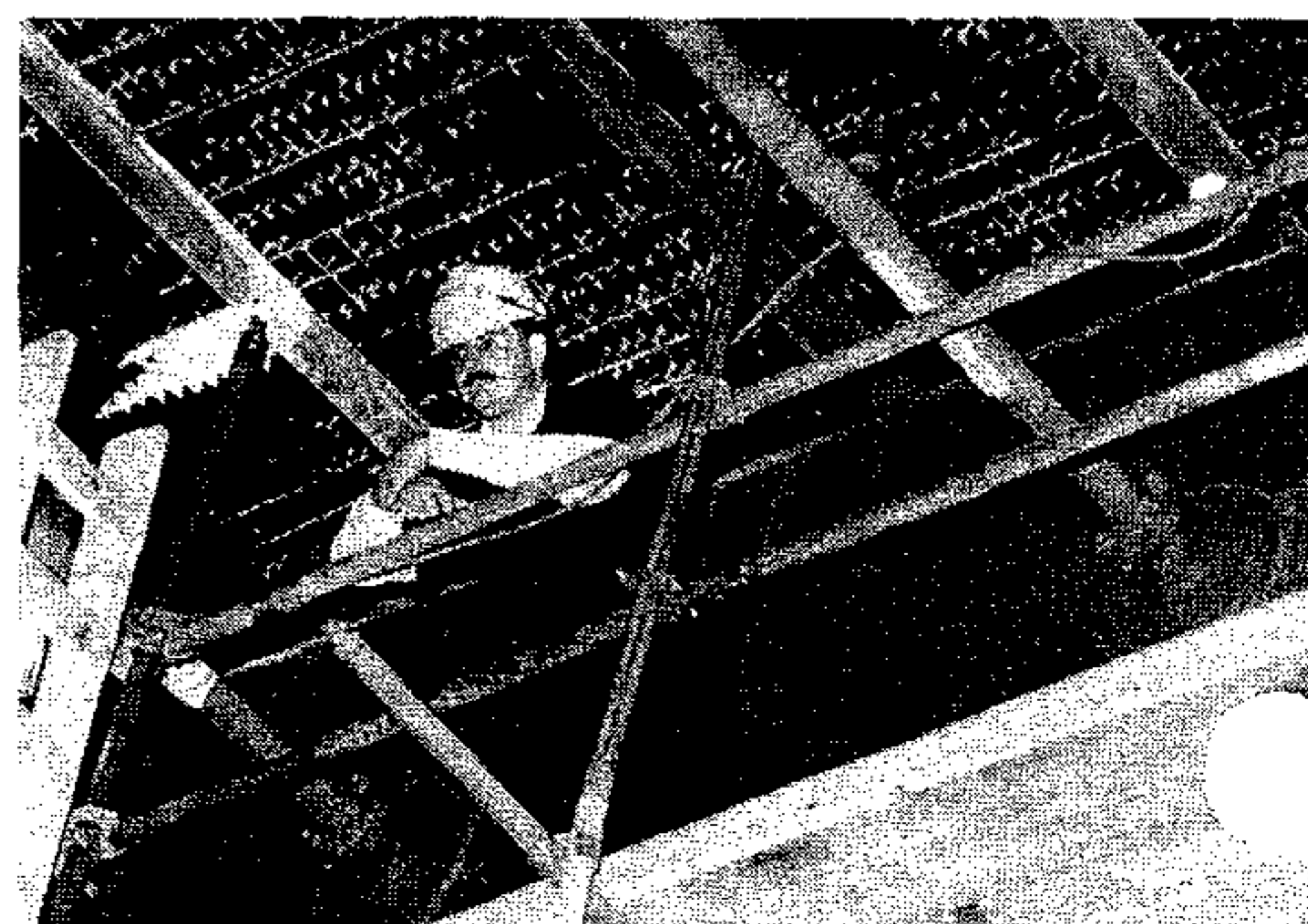
Views are of lower mist eliminators and spray headers at top of scrubber cell
