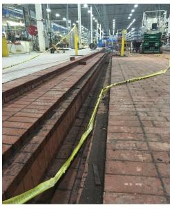
Atlastic 40 Membrane + Carbo-Alkor Mortar will provide excellent chemical resistance while the brick top will protect against thermal shock
