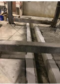
Anchor-Lok was delivered to the site in prefabricated sections, grouted into place, and placed into service within 5 days. The liner was specifically selected based on the chemical and temperature requirements we faced.
