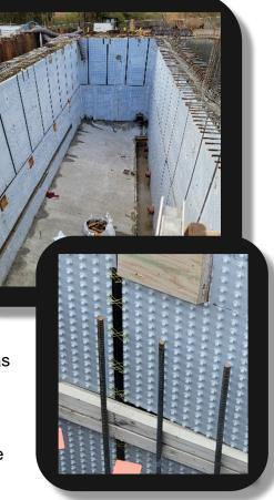
ANCHOR-LOK has excellent chemical, thermal and abrasion resistance and withstands external hydraulic pressure well in excess of a 100 ft. (30 m.) head pressure.
