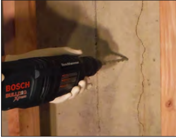
1. Drilling packer holes at a 45° angle towards the crack.
