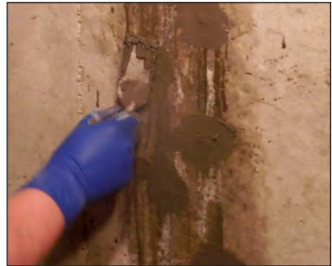
5. Sealing packer holes with Aquafin PLUG-IC after grouting.
