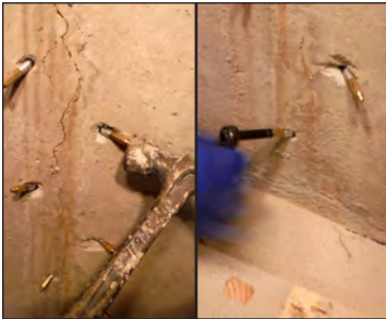
2. Inserting packer into the drill hole and tighten.
